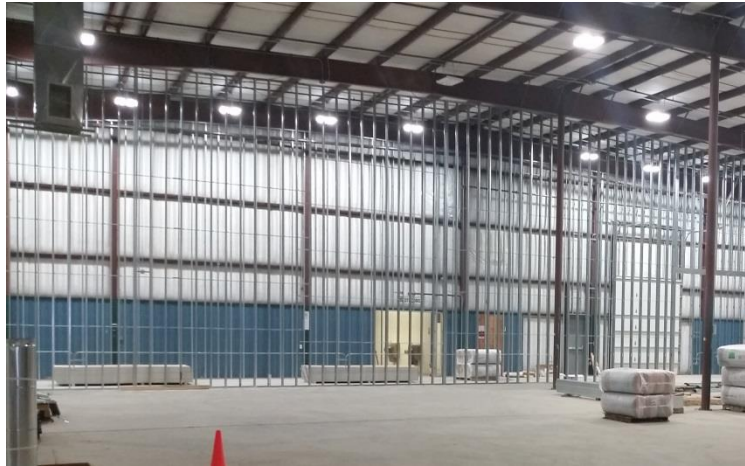
Preparing to create Clean Rooms
